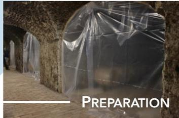
First step: Prepare the room and take the necessary safety measures. In practice, this means the blocking of all ventilation routes, which is easily achieved in most cases by sealing the doors or using plastic cover sheets.
